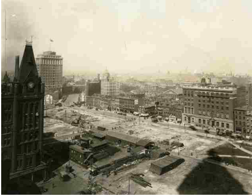
Figure 59. The entrance to the Parkway from City Hall Tower, c. 1915. The unimproved area where the commission successfully asserted their power over advertising is in the left center foreground (Fairmount Park Historic Resource Archive).
